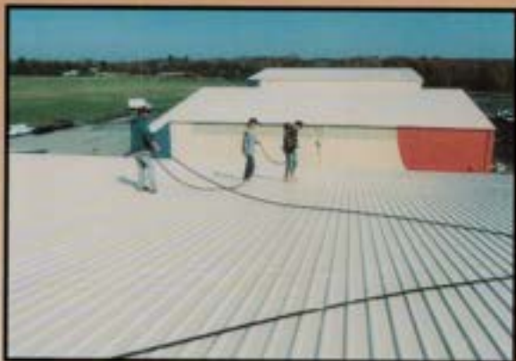
Final coat of Truco's Eterna-Seal® being applied resulting in a watertight membrane.
