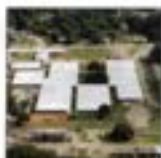
MEMORIAL ELEMENTARY SCHOOL ETERNA-SEAL® OVER METAL
